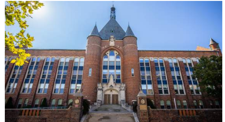
Image: Central Catholic High School's Main Building entrance and existing brick wall that runs along Fifth Avenue. The brick wall is proposed to be demolished and reconstructed. Fencing around the remainder of the site has also been proposed to improve the safety of students and staff on the urban campus.
