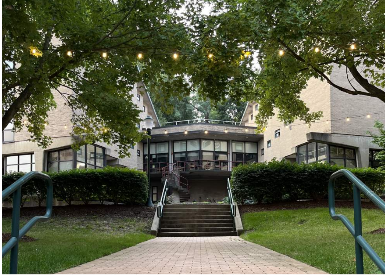
View of existing Hamerschlag House building through Boss and McGill courtyard.
