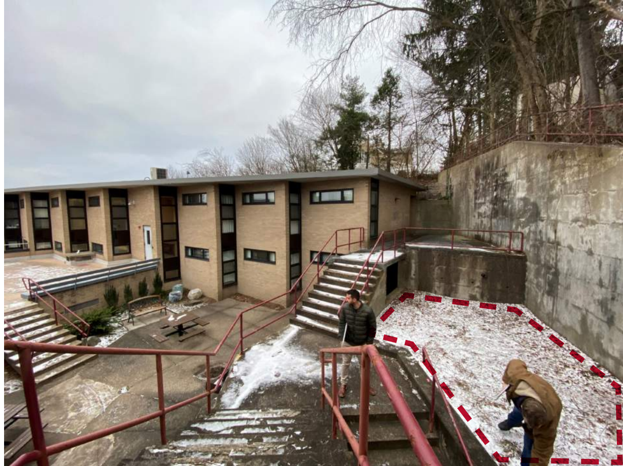
Proposed location of new Air Cooled Chiller with new concrete pad and acoustical enclosure
