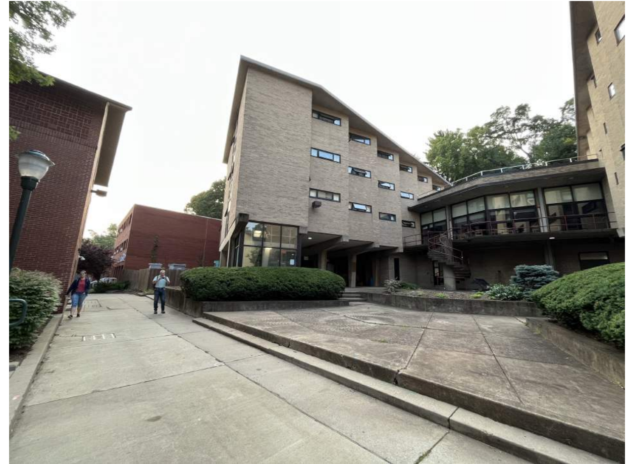
View of existing Hamerschlag House central patio and current fire lane access to remain
